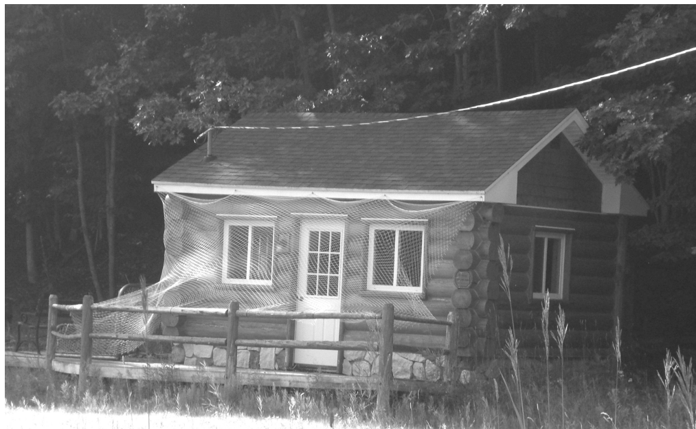
The new netting protects the windows from wanton discs.
